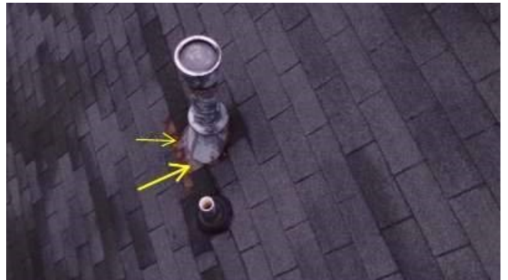
Photo 14-4 Required repair, replacement and/or evaluation
