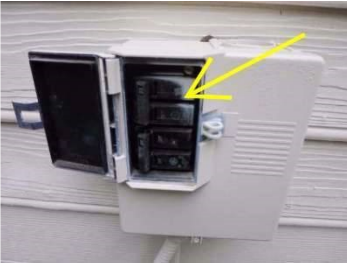
Photo 35-1 Paint on breakers!
