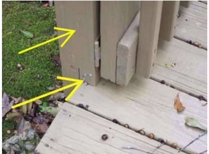
Photo 5-2 Rail loose needs to be repaired Recommend that a qualified person repair as necessary
