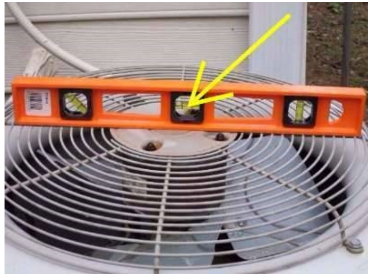
Photo 35-4 Not level needed repairs noted in this report should be brought to the attention of the contractor when it's serviced.
