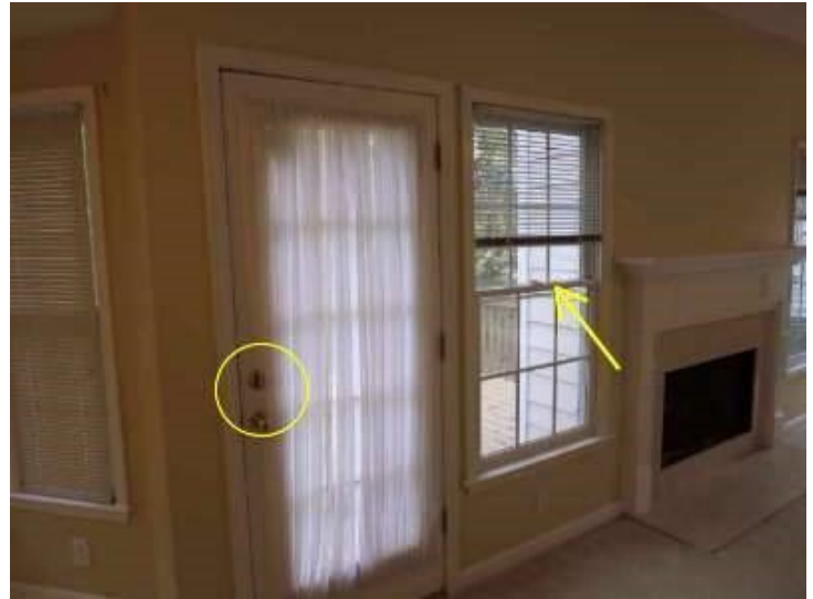
Photo 53-2 Dead bolt not latching, Window does not open freely
