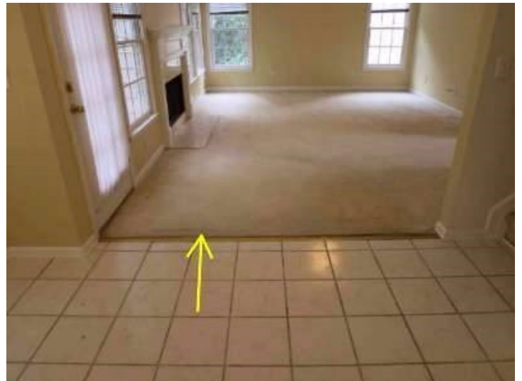
Photo 52-4 Trip hazard Recommend that a qualified person repair as necessary
