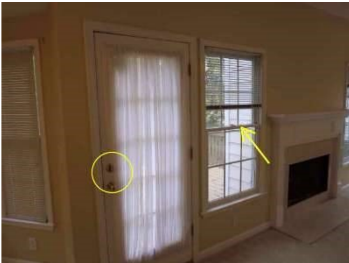
Photo 52-3 Dead bolt not latching, Window does not open freely
