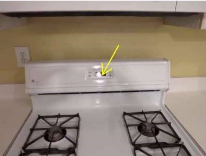
Photo 3-1 Display not functional Recommend that a qualified person repair as necessary!
