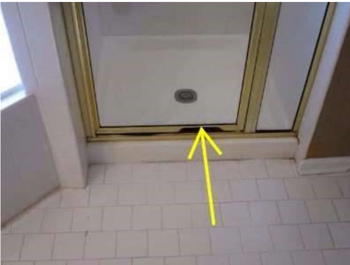
Photo X-17 Recommend that a qualified person repair as necessary
