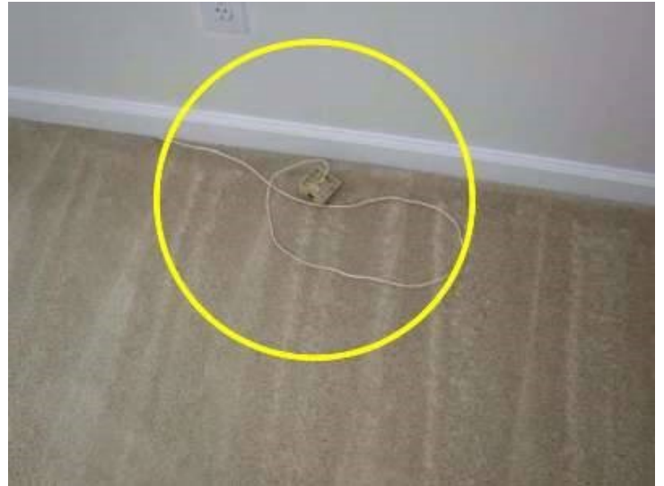
Photo X-16 Recommend that a qualified person repair as necessary
