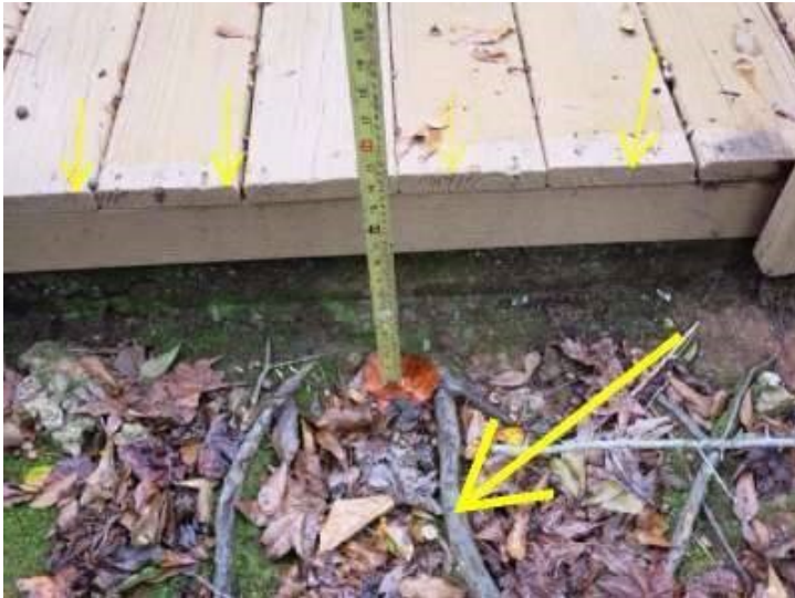
Photo 5-1 Needed repairs noted in this report should be brought to the attention of the contractor!
