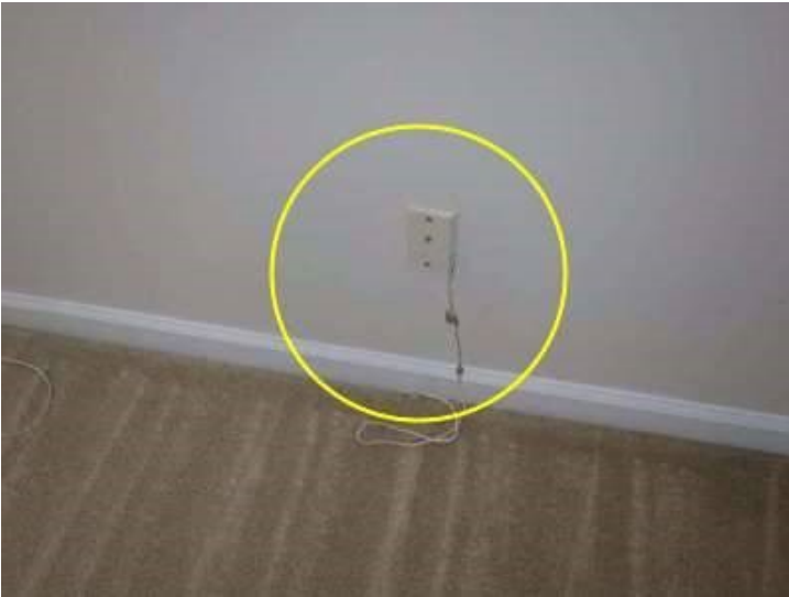
Photo X-15 Recommend that a qualified person repair as necessary
