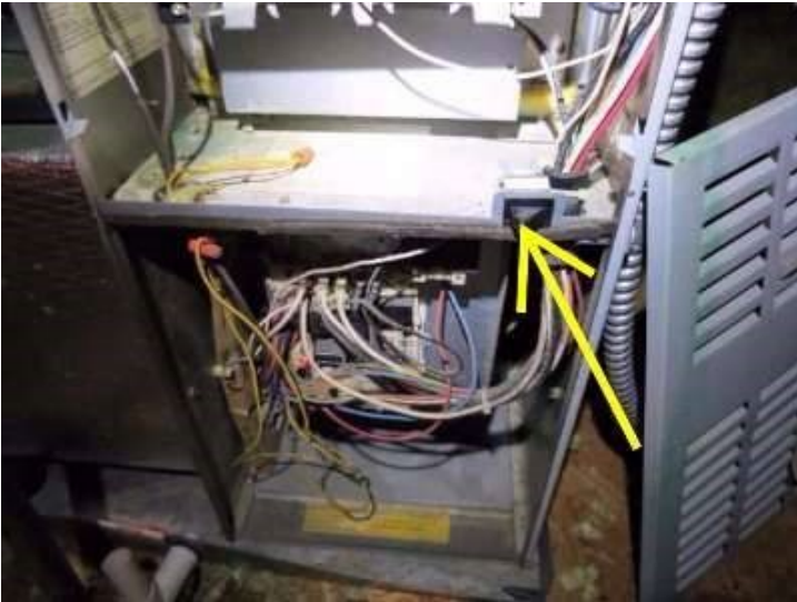
Photo 33-5 service switch need repairs ! needed repairs noted in this report should be brought to the attention of the contractor when it's serviced.
