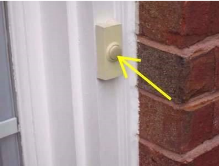
Photo X-11 Door bell is inoperable Recommend that a qualified person repair as necessary
